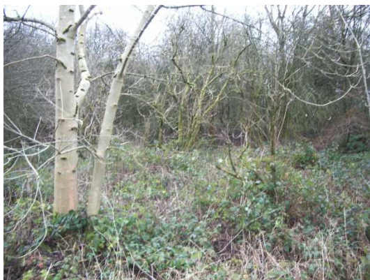
The south side of the rond-point submerged in brambles and trees. The bank at the back of the circular platform is just visible.
